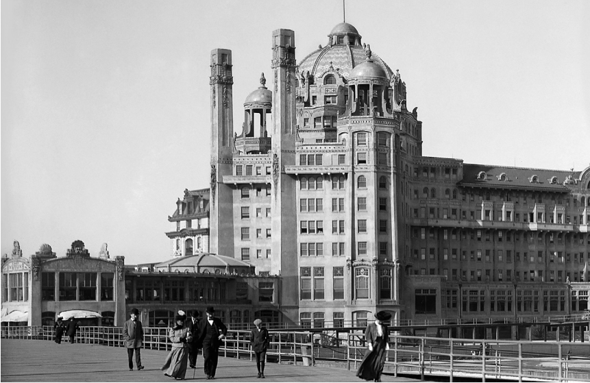
Figure 11: The Blenheim Hotel in Atlantic City, completed in February 1906, was constructed using the Kahn System of concrete reinforcement. (“Marlborough–Blenheim, Atlantic City, NJ,” circa 1908, Library of Congress Prints and Photographs Division, Detroit Publishing Company Photograph Collection: https://www.loc.gov/item/2016795897/ .)
