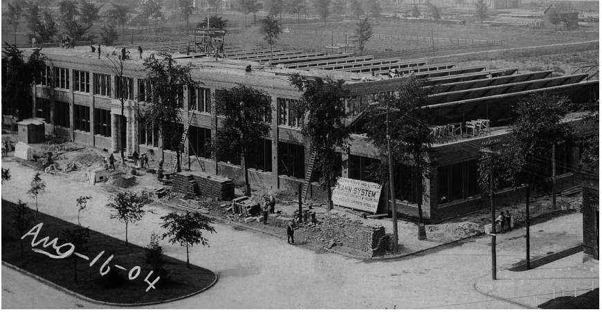
Figure 10: The headquarters and factory of American Arithmometer under construction on Second Avenue. The large sign propped against the front right side of the building reads, “Floors, roofs and lintels, Kahn System, Trussed Concrete and Steel Company.” (Courtesy of Charles Babbage Institute Archives, University of Minnesota Libraries, Minneapolis, MN—Burroughs Corporation Collection.)
